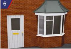
The bay window roof must be over flashed with lead flashing to the Lead Associations recommendations and on exposed sites a bead of sealant/lead adhesive is applied to avoid lifting the flashing.
