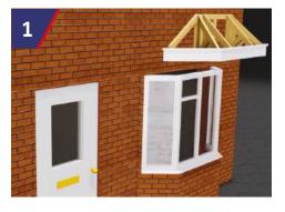
The GRP bay window roof is placed centrally onto the bay window. The bay window roof soffit should be level and large bay window roofs should have support props prior to fixing.
