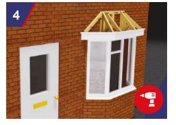
Once the StormFix Blue Fixing sleeves have been inserted into the holes, fully screw the StormFix 120 fixings into the sleeves.
