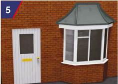
The window head is fixed to the GRP soffit using window manufacturers recommended fixings and sealed with suitable mastic joint.
