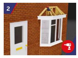
Using a 10mm drill bit, drill through the structural timber beam into wall structure at a maximum of 450mm centres, to suit the StormFix 120 Fixing.
