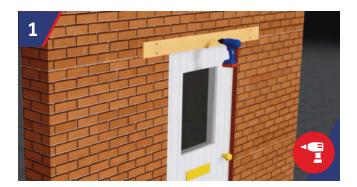
Position template central to the opening and the desired height. Using the centre of the 3 holes drill hole for fixing. Fix one side of template to wall, level up and repeat for other side of template.
