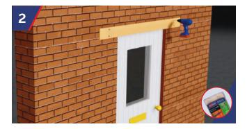
Usng a 10mm bit, drill holes to suit StormFix 80 Fixings using the 4 remaining pre-drilled holes as guides. Once all 4 holes have been drilled, unscrew and remove template.
