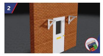
Once the StormFix Blue Frame Fixing Sleeves have been inserted into the holes, fully screw the StormFix 120 fixings into the sleeves. Conceal fixings using the bolt caps to cover the screws and plugs.
