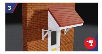
The canopy is placed on the brackets. Using a 10mm drill bit, drill through the GRP Upstand into wall structure at a maximum of 450mm centres, to suit the StormFix 80 Fixing.
