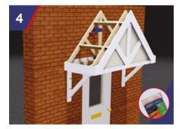
Insert StormFix Blue Frame Fixing sleeve 120 into the drilled holes.
