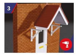
The canopy is placed on the brackets. Using a 10mm drill bit, drill through the GRP Upstand into wall structure at a maximum of 450mm centres, to suit the StormFix 80 Fixing.
