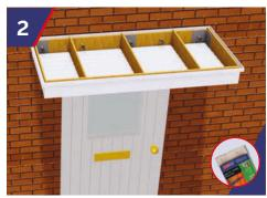
Insert StormFix Blue Frame Fixing sleeve 120 into the drilled holes. Once the StormFix Blue Fixing Sleeves have been inserted into the holes, fully screw the StormFix 120 fixings into the sleeves.
