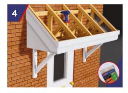
Insert StormFix Blue Frame Fixing sleeve 120 into the drilled holes.
