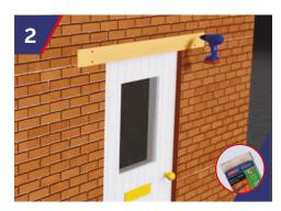
Using a 10mm bit, drill holes to suit StormFix 80 Fixings using the 4 remaining pre-drilled holes as guides. Once all 4 holes have been drilled, unscrew and remove template.
