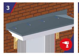
Insert StormFix 80 into the drilled holes. Ensure the canopy is level and maintains a fall to the front.
