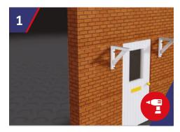
The Gallows Brackets are fixed into the wall in two places ensuring the gallows are level. Using a 10mm drill bit, drill into wall structure, to suit the StormFix 120 Fixing. Insert StormFix Blue Frame Fixing Sleeve 120 into the drilled holes.
