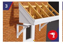
The canopy is placed on the brackets. Using a 10mm drill bit, drill through the rear structural timber truss into wall structure at a maximum of 450mm centres, to suit the StormFix 120 Fixing. Top and bottom rail running canopy length to be fixed back.
