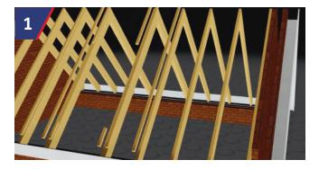
Trimming rafters to be positioned under side cheeks with outer edge of outer most trimmer in line with GRP side cheek. Trimmers
