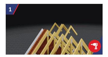
Fix support noggins to the inside of the rafters and insert external quality plywood panels between the rafters ensuring top of plywood is level with top of rafters.
