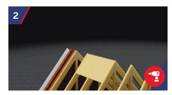
Screw fix the plywood panels to the noggins at a maximum 150mm centres and with minimum of 8 screws. It is imperative the plywood is securely fixed as the plywood will act as the main fixing point for the chimney.
