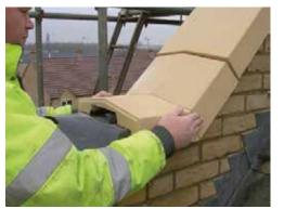
Clip on pre mitered sections and stop
