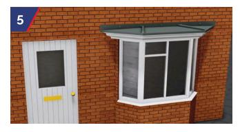
The window head is fixed to the GRP soffit using window manufacturers recommended fixings and sealed with suitable mastic joint.
