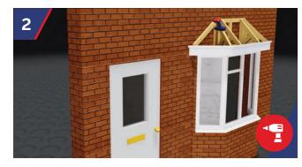
Using a 10mm drill bit, drill through the structural timber beam into wall structure at a maximum of 450mm centres, to suit the StormFix 120 Fixing.
