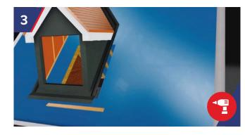
Fix timber cocking fillet to support lead. Lift GRP Dormer into place onto roof. Timber fillet can be positioned at a later date if the roof isn't being finished at the same time as the dormer installation.
