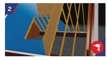
Fix 18mm plywood support between rafters. Ensuring the plywood is the same height as the top of the truss line. Fix roofing felt to roof. Only the area under the dormer needs to be felted during the lifting and fitting of the dormer.
