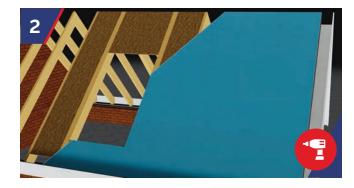
Fix 18mm plywood support between rafters. Ensuring the plywood is the same height as the top of the truss line.
