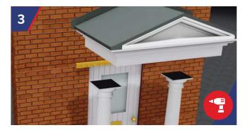
The Portico is placed on the columns, and the tops of the columns are screw fixed to the soffit of the portico. The soffit is screw fixed to the wall plate at 450m centres.
