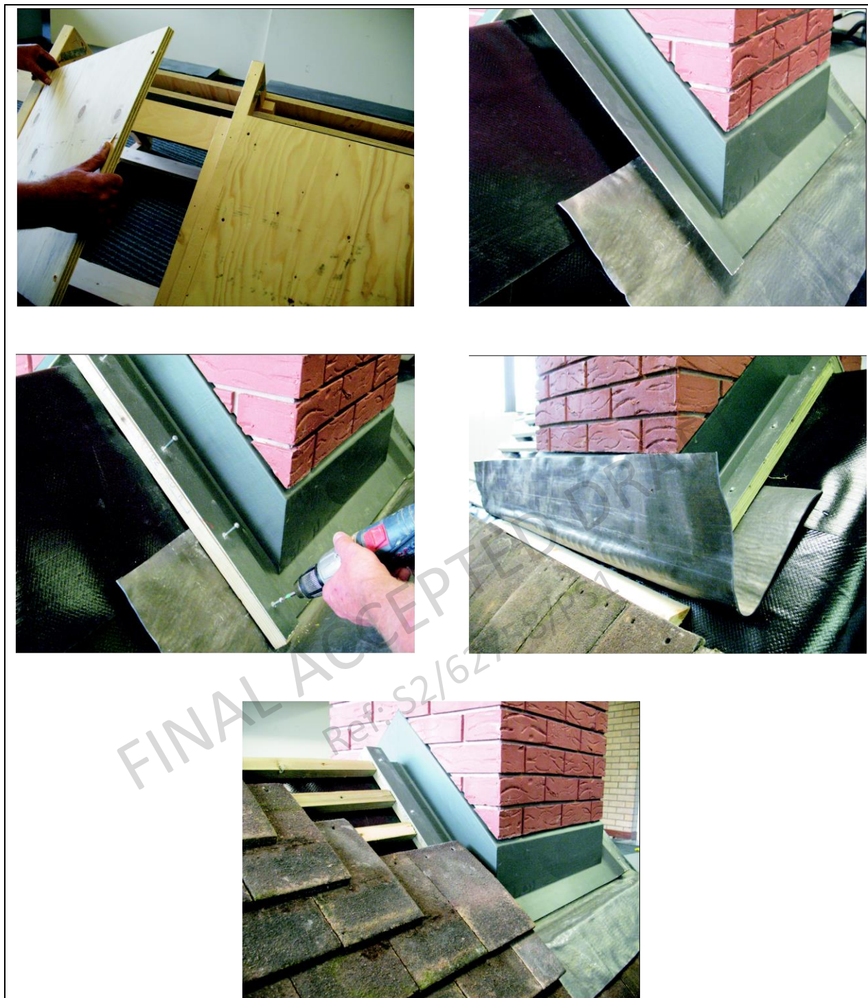
Figure 2 Method of installation
